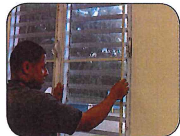
Install or repair window & door screens.
