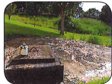
Keep septic tanks sealed.
